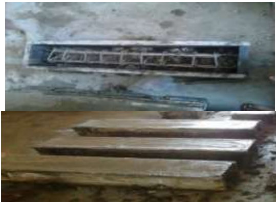
Fig 9.6 Casting of beams
